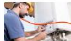
Gas / Oil Burner
